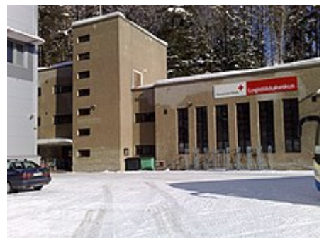
The Logistics Centre of the Finnish Red Cross in Tampere, Finland
