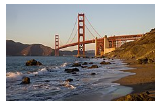
Bridges, such as Golden Gate Bridge, allow roads and railways to cross bodies of water.
