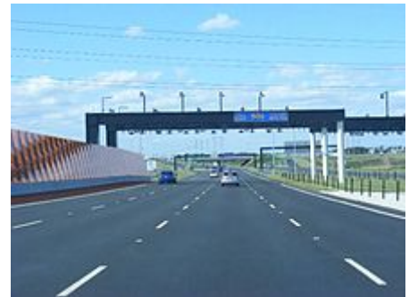
Eastlink - Wellington Rd Northbound Toll Gantry
