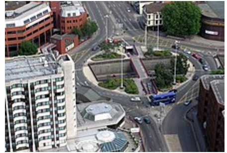
The engineering of this roundabout in Bristol , United Kingdom, attempts to make traffic flow free-moving.
