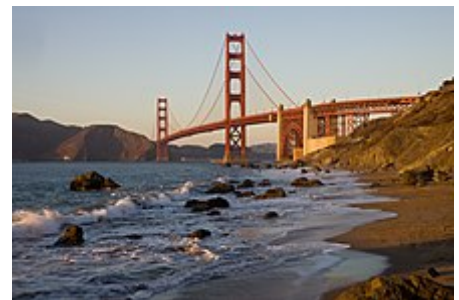
Bridges, such as Golden Gate Bridge , allow roads and railways to cross bodies of water.
