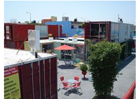
Container City in Cholula , Mexico uses fifty old sea containers for 4,500 m 2 (48,000 sq ft) of workshops, restaurants, galleries, etc., as well as some homes.
