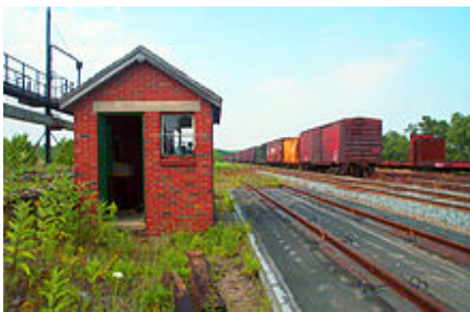
Bulk freight car scales at the MMA Mack Point yard, Searsport, Maine
