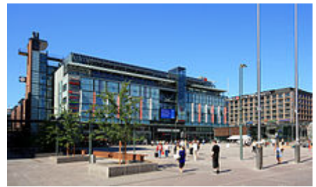
Underground bus and coach terminal and metro station are located underneath the Kamppi Center in Helsinki, Finland
