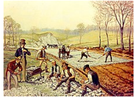
Construction of the first macadamized road in the United States (1823). In the foreground, workers are breaking stones "so as not to exceed 6 ounces in weight or to pass a two-inch ring". [12]
