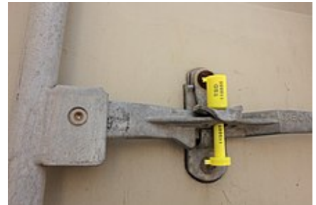
Tamper seal on the door locking bar handles of an ISO container
