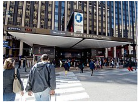
Penn Station in Midtown Manhattan, New York City , the busiest transportation hub in the Western Hemisphere
