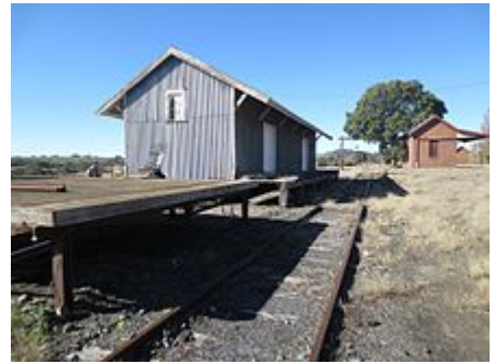
Typical small transshipment station platform and warehouse - rail to road transport (abandoned) (2016)
