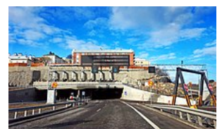
Tunnels, such as the Tampere Tunnel, allow traffic to pass underground or through rock formations.
